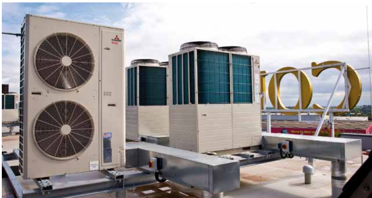
High-tech climate for big properties: comfort air conditioning system Mitsubishi Heavy industries KX6.
