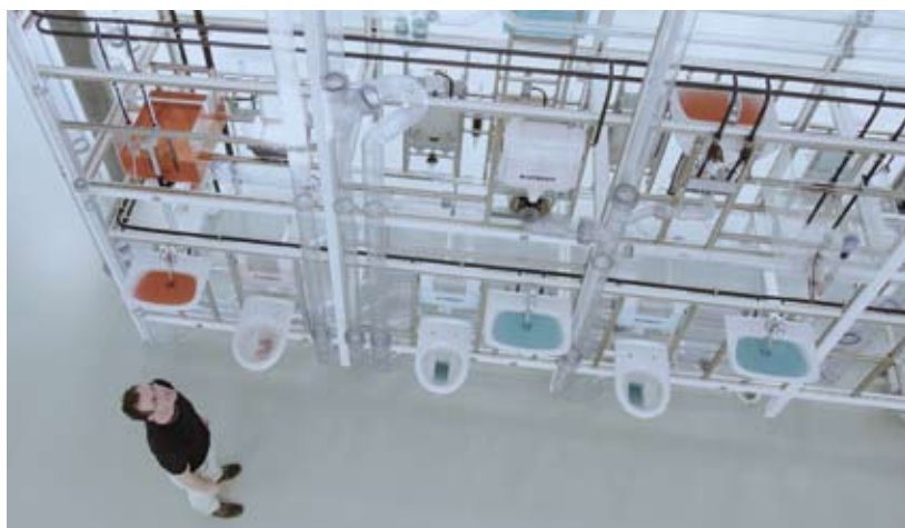
The Geberit test tower is a demonstration and testing system helping the company identify, visualize and solve potential sanitary problems.
